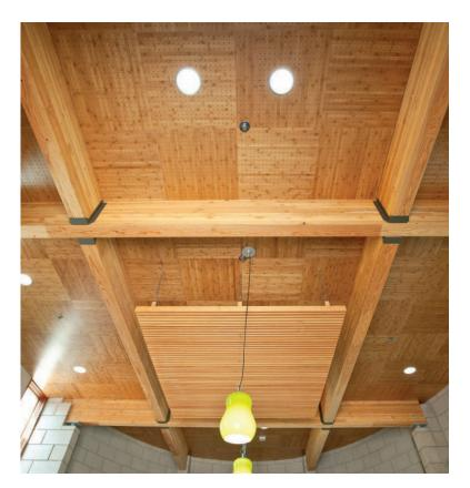
Madrid's **wood ceiling tiles** are manufactured with class A fire rated cores with particle board or medium density fiber board (MDF). Our tiles are manufactured with 100% post-consumer recycled content and contain no urea, formaldehyde or VOCs.
